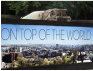
Bristol building works Bristol Construction work
