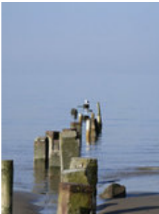
Gull on Concrete post gull on post
