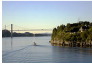
Norway bridge over fjord with...
