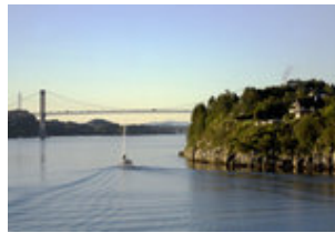
Norway bridge over fjord with...
